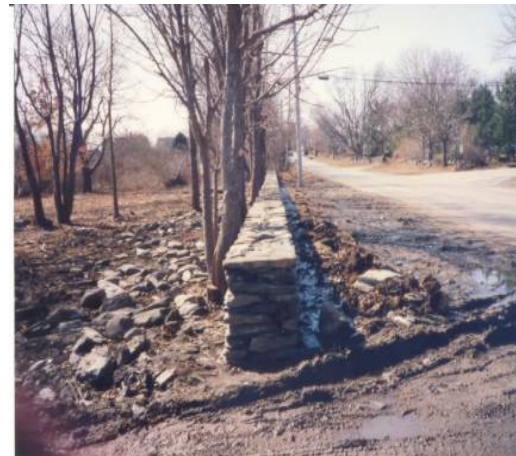
Paradise Valley Park stone wall under construction, Spring 1993.
